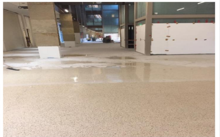
• Concourse- Terrazzo Phase 4 (Atrium)
