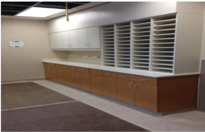
• Energy Center- Office Area Casework Installation
