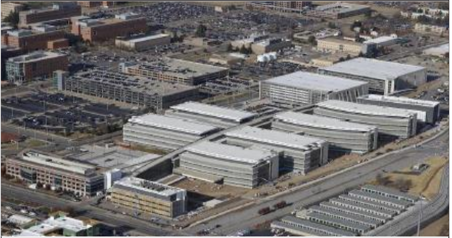
Aerial of the full site facing northeast taken on December 1, 2016.
