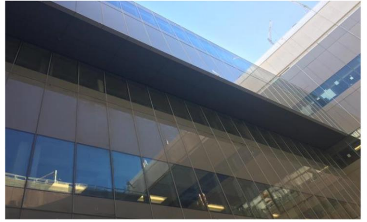
• Diagnostic and Treatment Building – Courtyard Soffit
