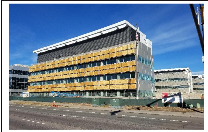
• Research – Solar Tube Installation Complete
