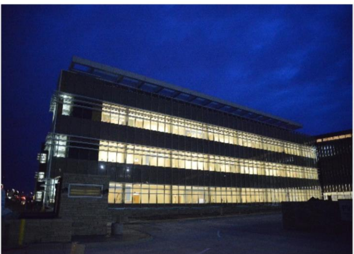
• CBC – South Elevation of Curtainwall
