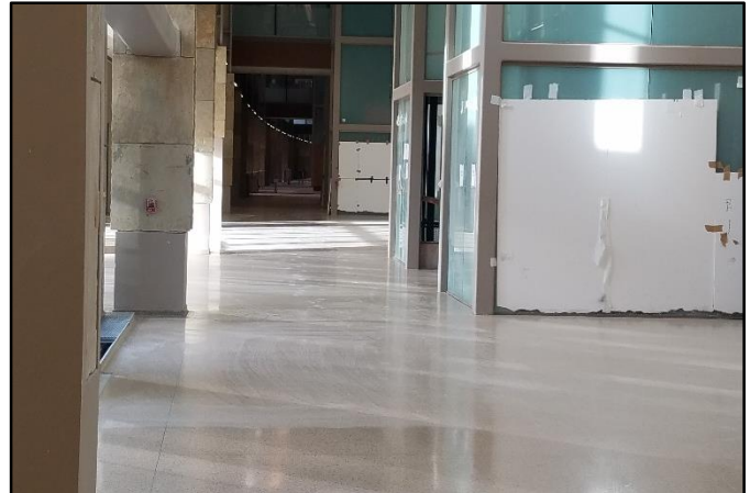
• Concourse- Terrazzo Finish (Atrium)
