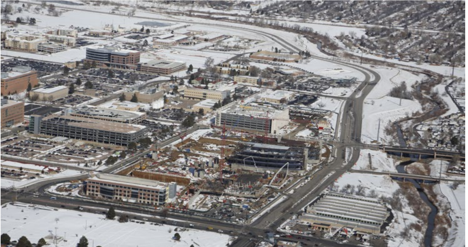
March 1, 2013 Aerial of the full site facing north.
