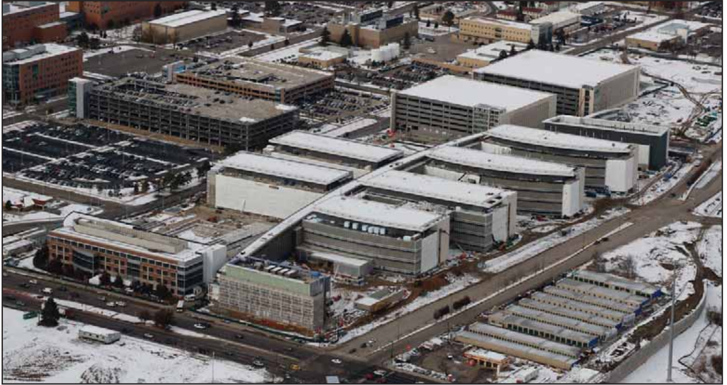
Aerial of the full site facing northwest taken on December 1, 2015.
