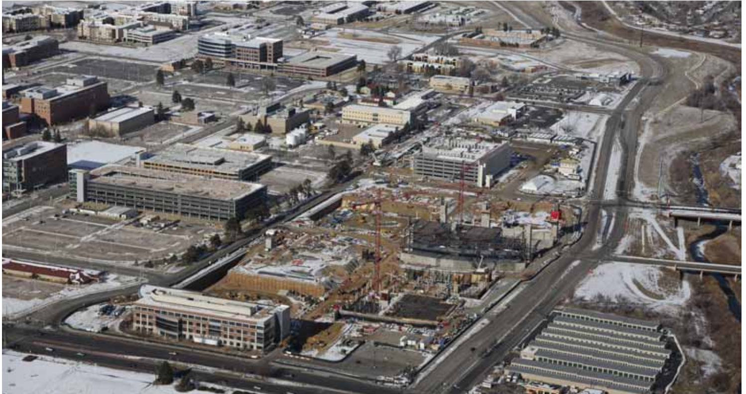
January 2, 2013 Aerial of the full site facing north.
