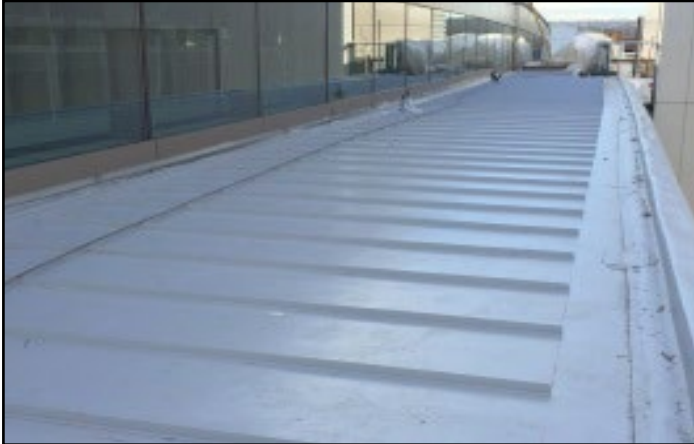
Concourse high roofing membrane installed.
