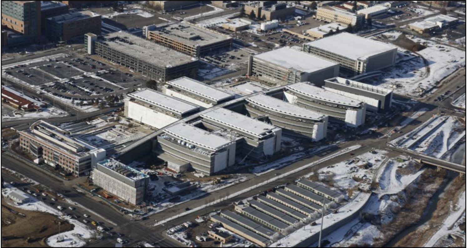
Aerial of the full site facing northwest taken on January 4, 2016.
