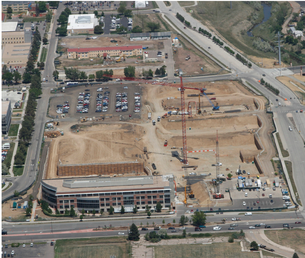
5-17-12 Aerial of the full site facing north.
