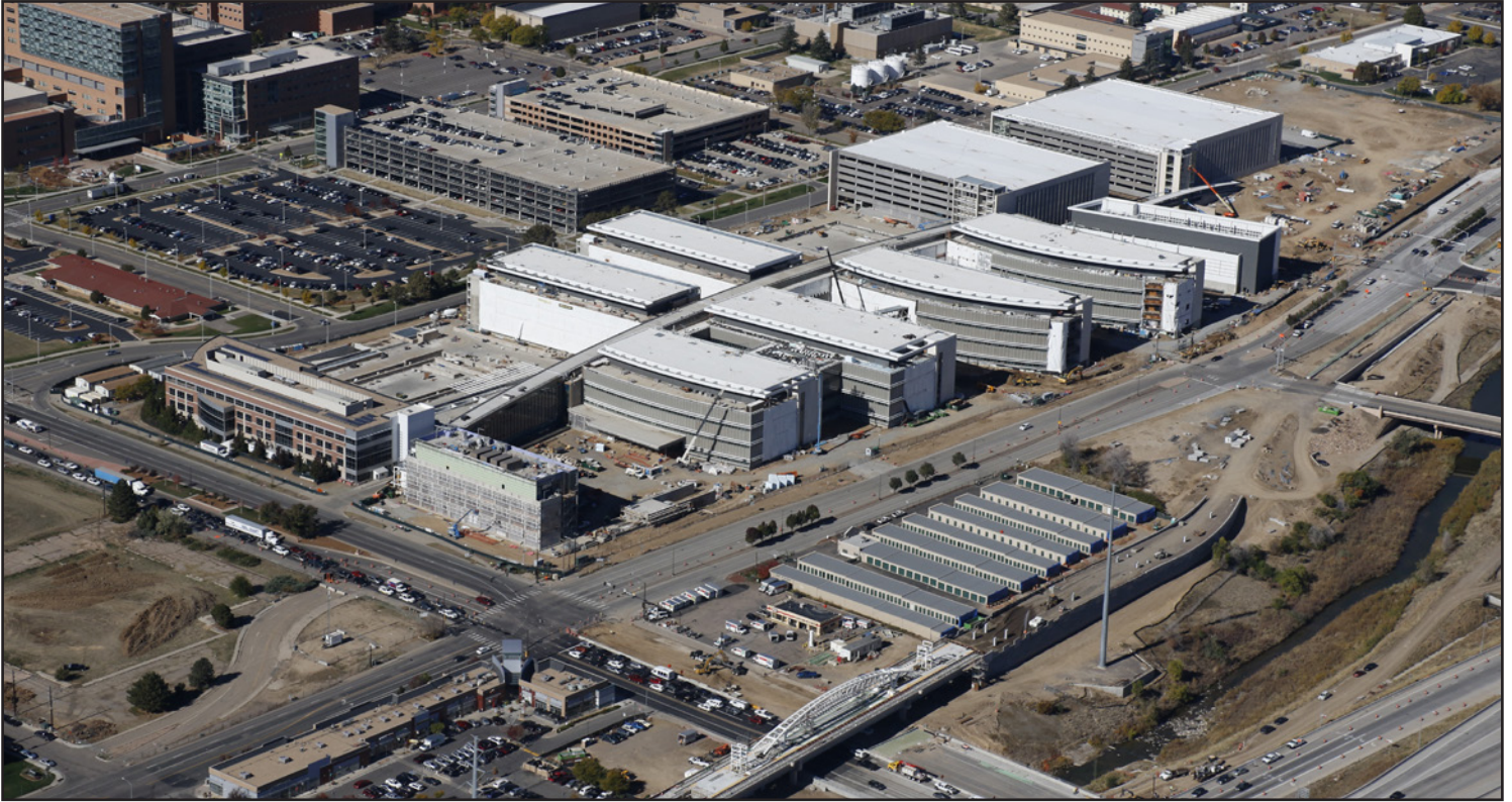
Aerial of the full site facing northwest taken on November 1, 2015.
