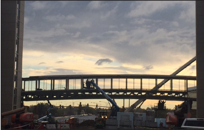
Exterior framework for cladding in progress on the Concourse pedestrian bridge.
