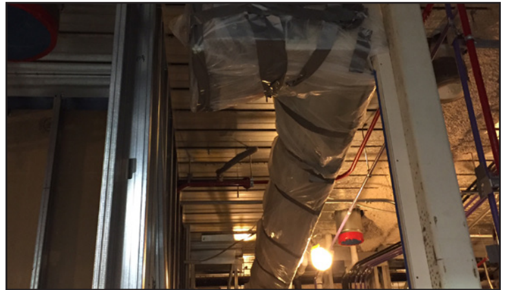
Lighting boom equipment installed in the Emergency Room on Level 1 of the Diagnostic and Treatment Facility.
