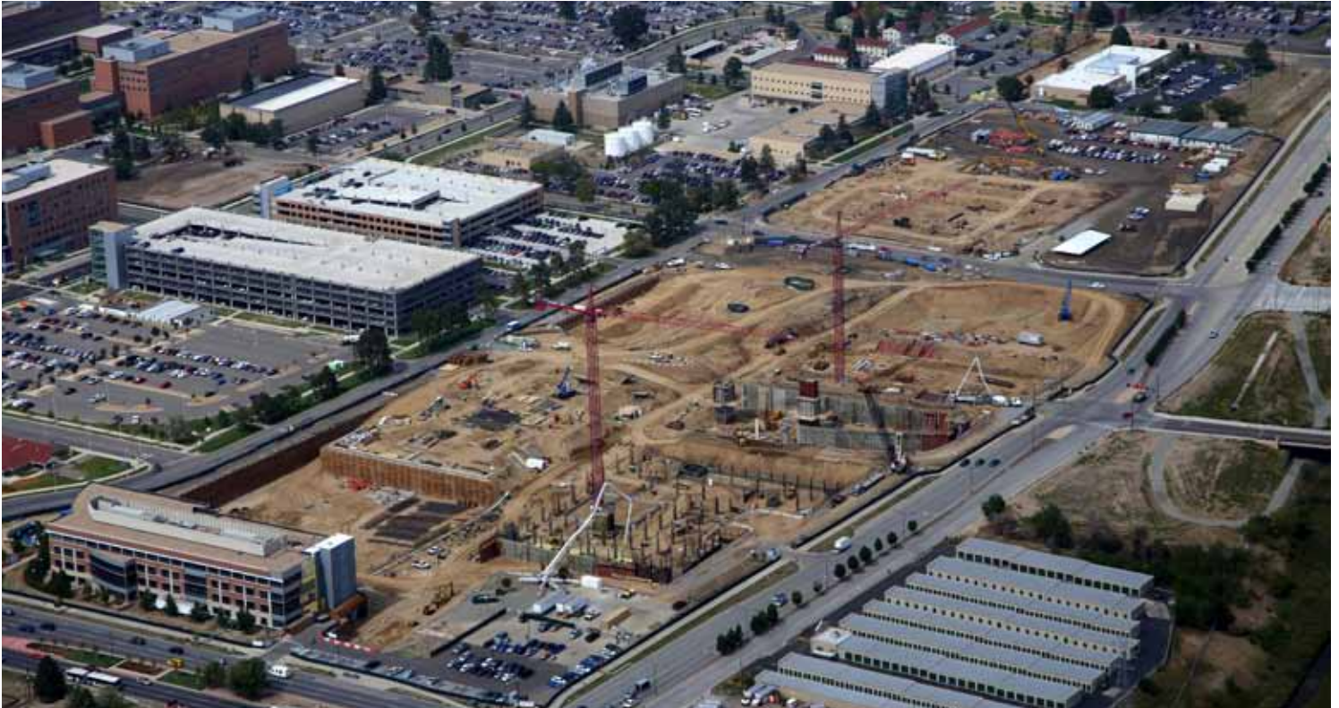
September 21, 2012 Aerial of the full site facing north.
